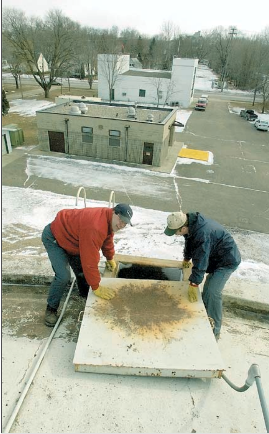
Dennis Duchene, superintendent of Faribault's water department, left, and foreman Jim Hausen look inside the water reservoir at the Faribault Water Works Station on Monday. Behind them are the chemical feed building and the pumping station. (Kelli Wencil / Daily News)
