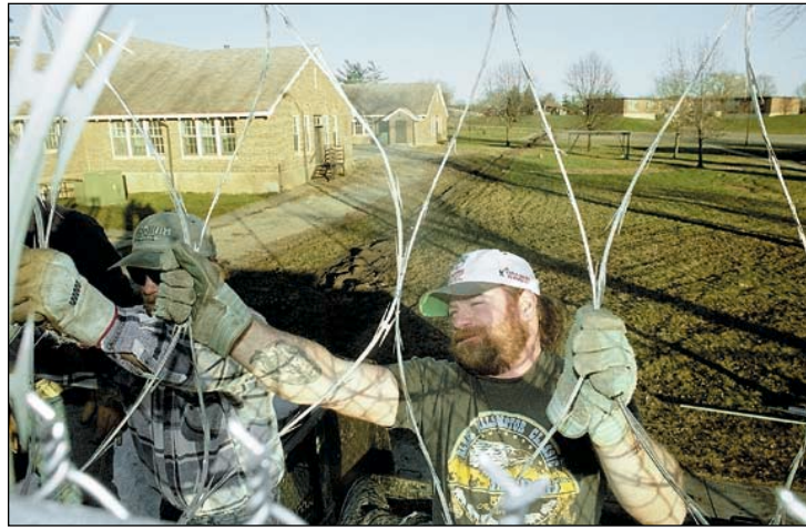
Keith Finley, right, and Kevin Horsman attach wire razor ribbon to a fence at the Minnesota Correctional Facility-Faribault during an expansion of a minimum-security area in 1998. The prison has proposed a new expansion. (File Photo / Daily News)
